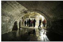
Photos by Gregory Rice/Staff Photographer This arched area will be part of the fitness room in the basement of The Mill at Saco Falls, a $14.4 million project converting a 165-year-old building originally used by Laconia Manufacturing Co. into 66 apartments. A tour of the 80,000-square-foot property took place Monday.
